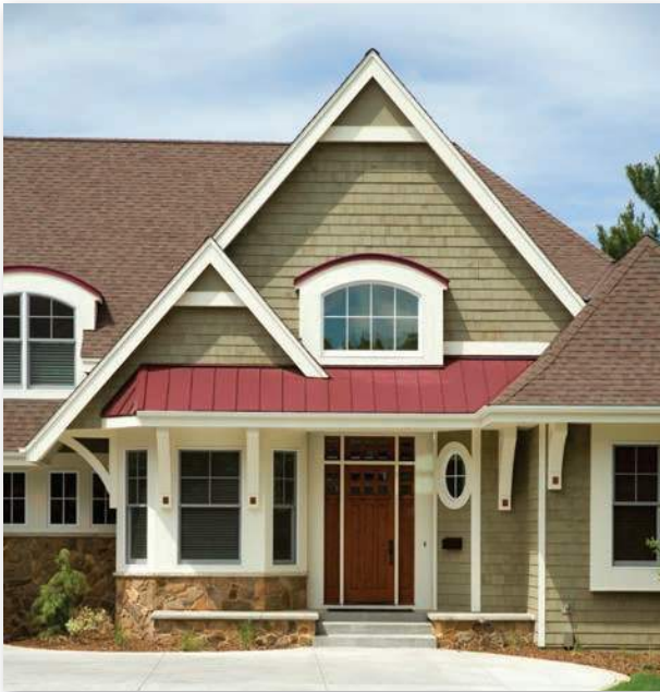
Consider using 1x and 2x board sizes to add detail to fascias and window casing treatments.
