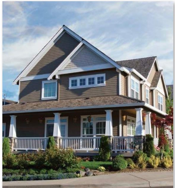
Trim boards complement other architectural details on this Craftsman/bungalow style house design.
